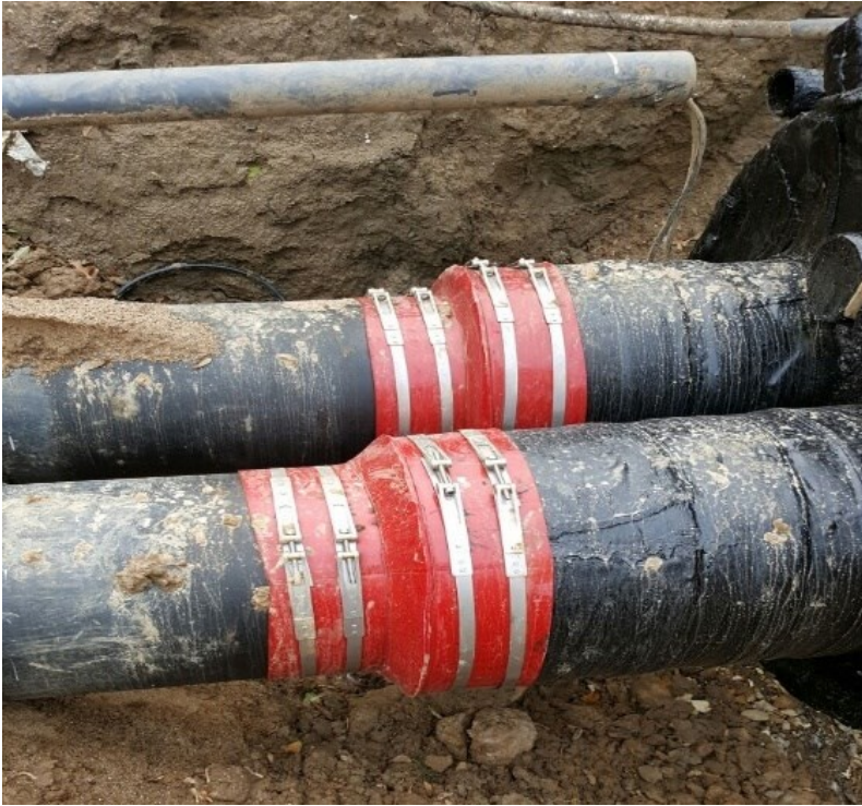
Figure 95, KMR-Sealing sleeve pipe to casing pipe with heavy-duty steel straps
