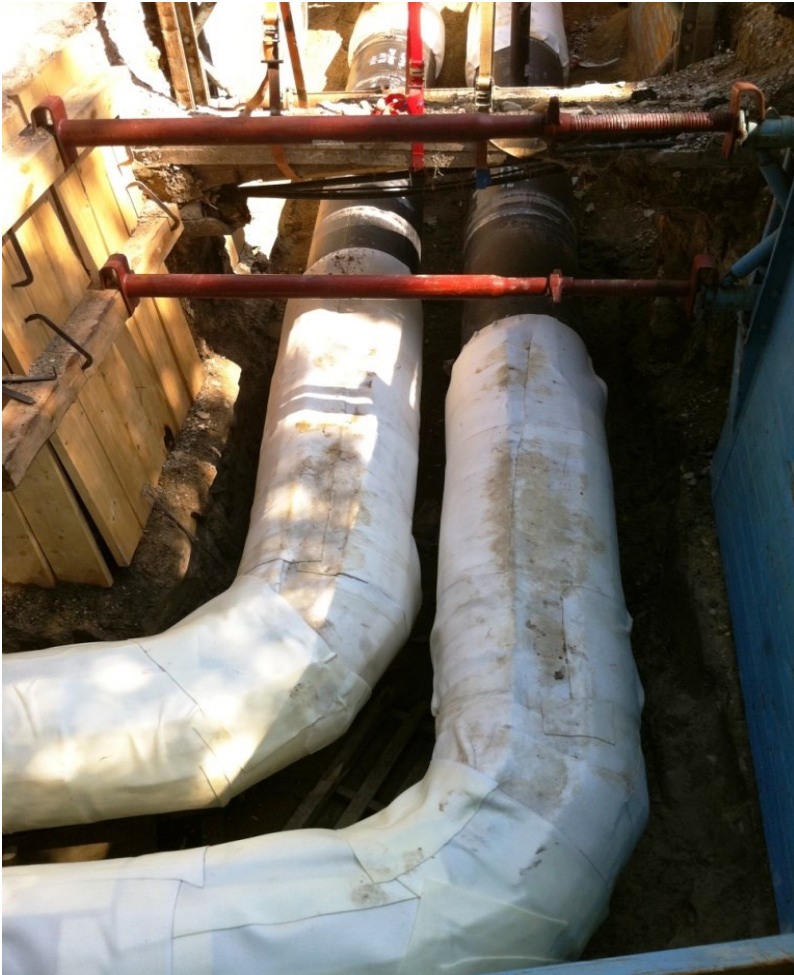
Figure 84, Single-ply cushioning with full encasement
