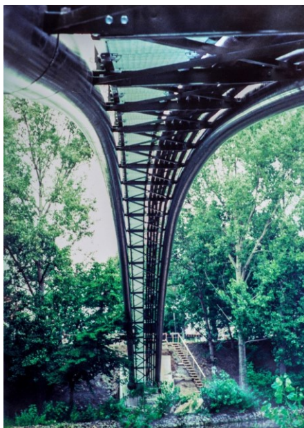
Figure pipe bridge with steel casing pipe
