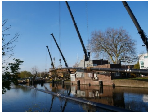
Figure: trenchless laying Horizontal Directional Drilling
