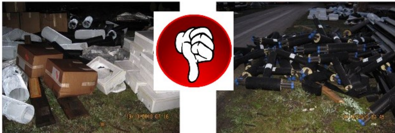
Figure 30, Improper storage
