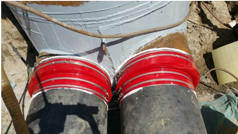
Figure 94, Example of a (KMR) Pre-insulated Pipe structure insertion
