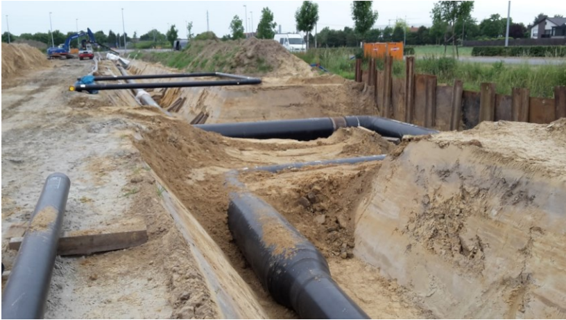
Figure: U - bend with casing pipe extension
