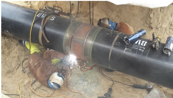
Illustrations: Building connection with half shells
