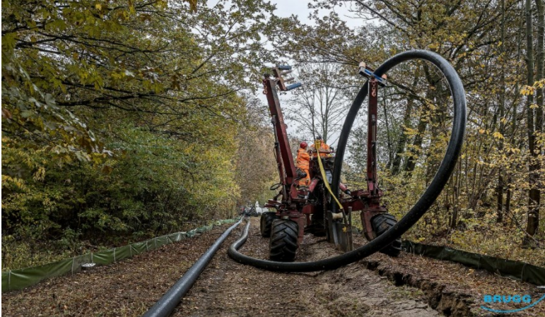
Plowing in with flexible steel casing pipes. Image source: Image X21.de-ReinerFreese
