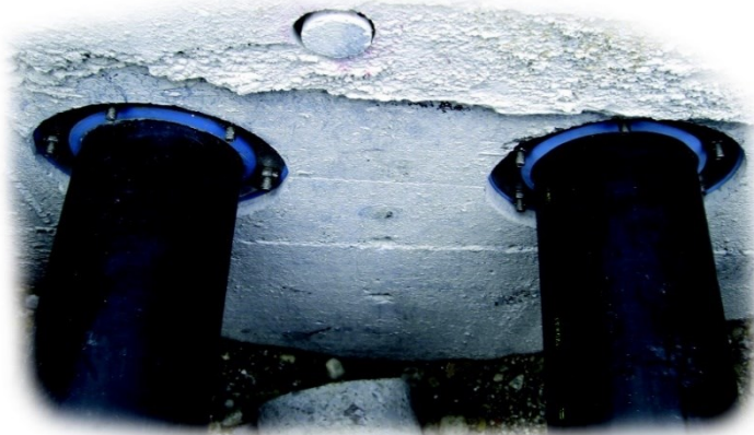
Figure 89, Example of house connection with Pressio FW
