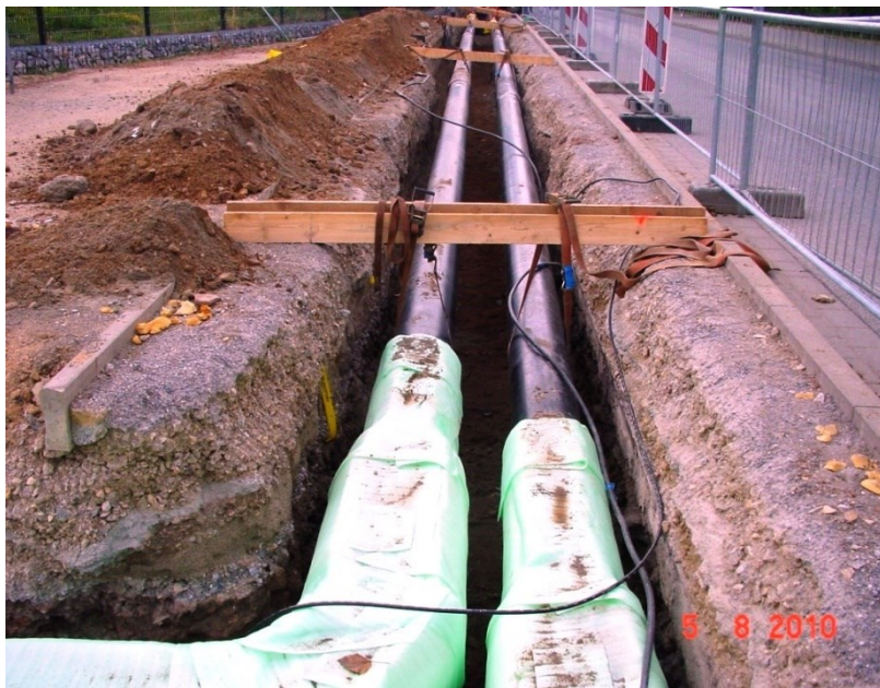
Figure 83, Multilayer oval-shaped padding of an L-leg with full wrap.
