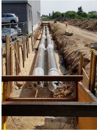
Figure SMR - Construction units in the pipe trench
